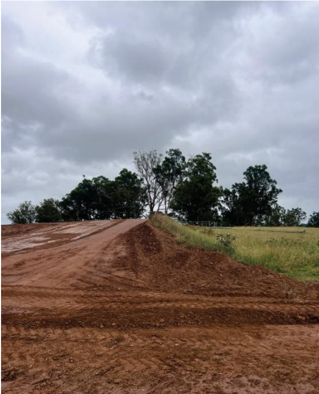
Picture 1 Standing on the future Road 14 looking north
